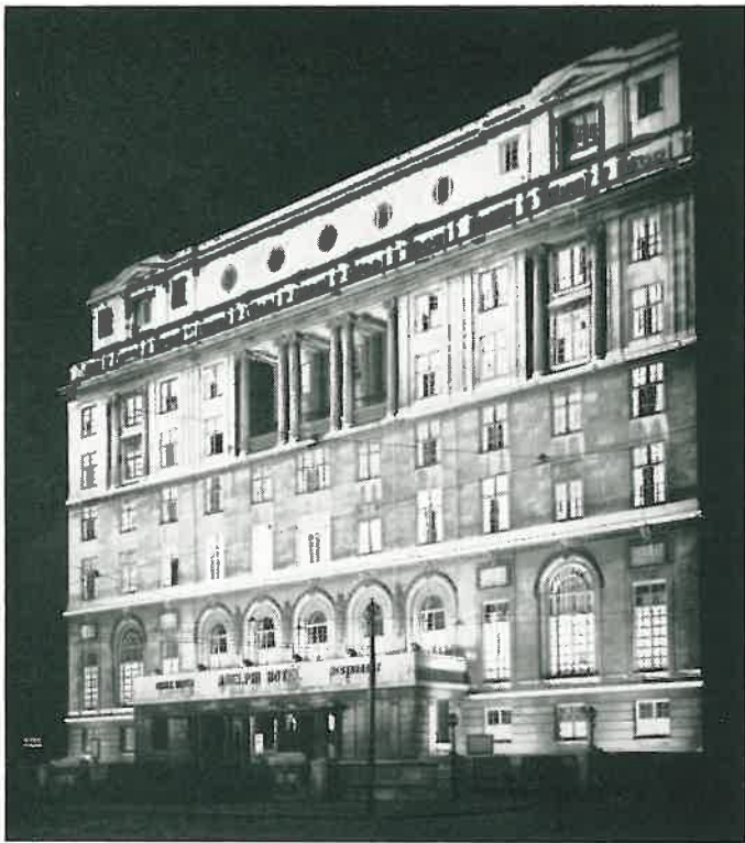
An early BTH mercury discharge floodlighting installation using Type F 'Mercura' projectors at the Adelphi Hotel, Liverpool.
