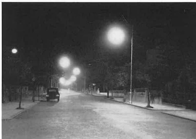
An early streetlighting installation using horizontally burning mercury lamps in experimental Mazda fittings.
